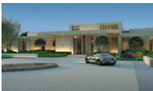
VIP Majlis for HH Sheikh Mohammed bin Rashid Al Maktoum, Dubai
